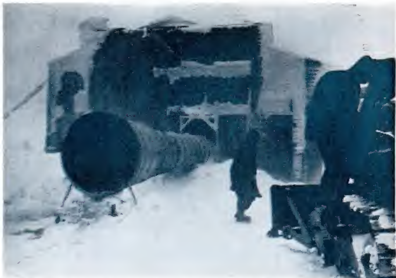
Exit end of wind tunnel juts from icing-research hangar at summit. Savage weather is ideal for test purposes
